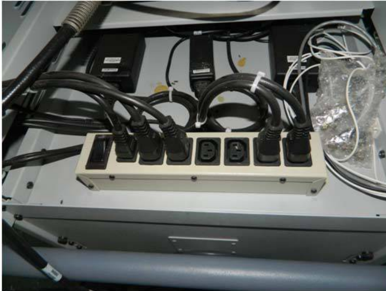
Fig. 7: Power strip on the vision cart
