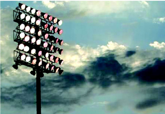
Fig. 2.6: A metal halide gas discharge lighting system provides illumination for a college baseball game. Note the various colors of the lights as they warm up
